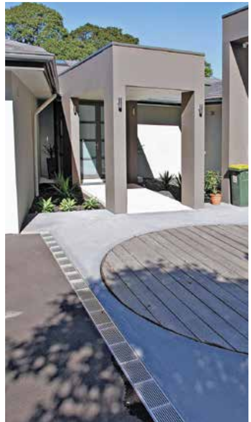
HDGLS-6S Heavy Duty Aluminium Grate in a residential driveway application.
