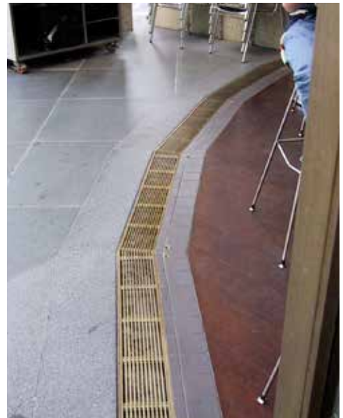
BRGNS-8S Solid Brass Trench Grate site segmented to create curve, this product could have been supplied factory curved if required.
