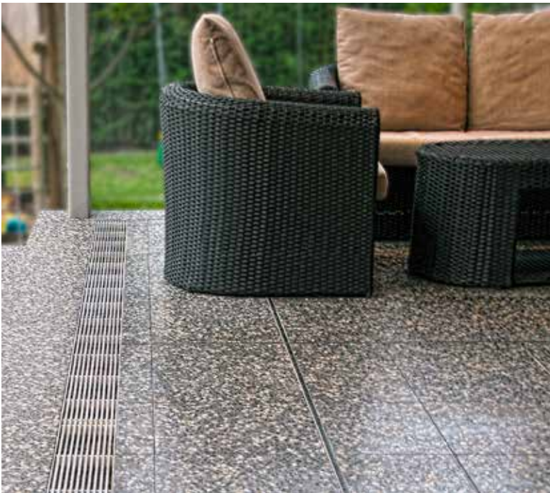
ALGLS Series installed in a modern terrazzo floor in an outdoor entertainment area.
