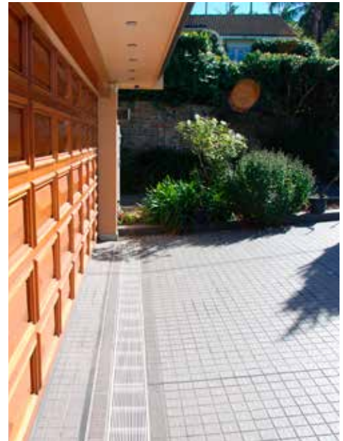
HDGLS Series installed in a residential driveway application.
