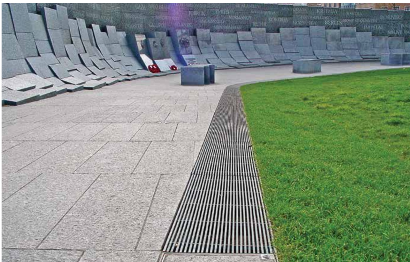
Australian War Memorial, Hyde Park Corner, London. Brass grates specially patinated to appear aged. Photo above: Grate segmented to create curve. This product could have been supplied factory curved on request.
