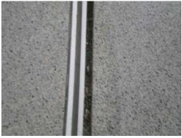
Mastic has disappeared eventually the recess will fill with dirt and debris and thermal expansion of the structure is likely to cause the cover to rip off.
