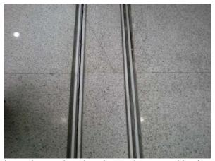
The following pictures show where the sealant has been depressed by foot traffic causing it to de-bond, this will also cause issues overtime and will eventually cause the cover plate to lift.
