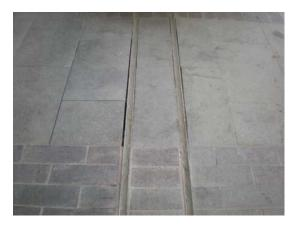
Both the Latham details that follow address this issue, which is generally caused by the fact the structural expansion joint covers are move more that a sealant type joint will allow causing bond failure, this combined with the problems associated with the sealant depressing over time and causing trip hazards and unsightly dirt traps, has prompted Latham to offer their PAVA Series.
