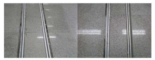
The final images shows extreme damage to the paving, this is caused general by the cover plate being to thin for the application and deflection occurring, also it is unlikely a suitable high strength non shrink epoxy bedding compound has been used under the expansion joint cover. In the second lot of photo's
