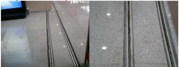
These pictures shows the sealant failing badly under minimal movement, causing trip hazards, hygiene issues.
