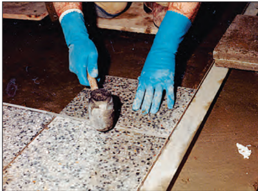
3. The floor finish and Loc® Strip can then be levelled to the required height.
