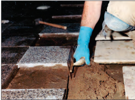
1. The installer makes a trowel cut in the bed through to the slab ensuring it is as wide as the neoprene insert and free of debris.
