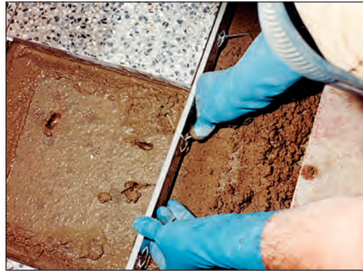
2. The installer then inserts the Loc® Strip, working into the bed to the required depth. At this stage the installer inserts the wire anchors, ensuring no debris gets under the Loc® Strip.
