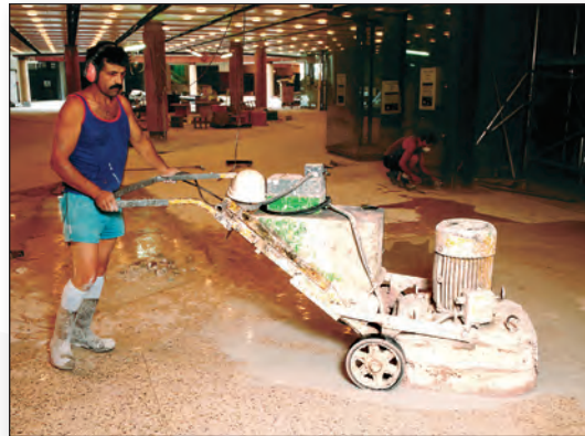
4. Loc® Strips 31mm or deeper can be ground insitu.
